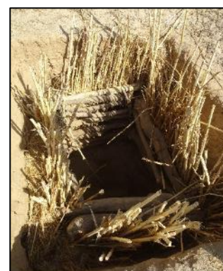
Figure 9. A hand-dug well lined with crop residue and wooden poles
