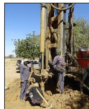
Figure 10. Drilling of a borehole
